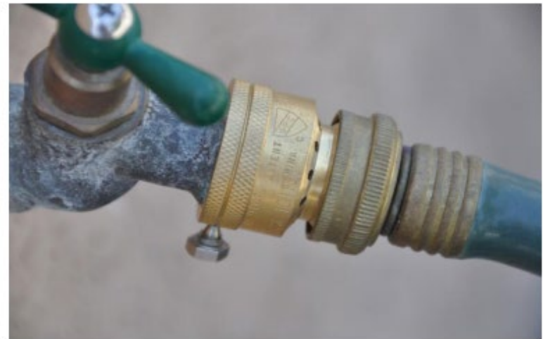
Hose bib backflow preventer placed on a backyard hose.
